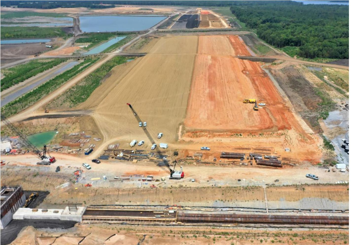
Bois d'Arc Lake Dam and Reservoir Aerial When complete, the dam at Bois d'Arc Lake will be 2-miles-long and 90-feet-tall at its highest point. The brown-colored dirt will be the water-side of the dam. The two conduit pipes that will transport water from the intake tower to the raw water pump station are visible in the lower portion of photo. **Buy I**
