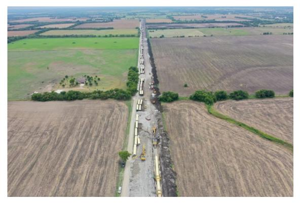
Crews are busy stringing and placing raw water pipe to deliver the water for treatment.
