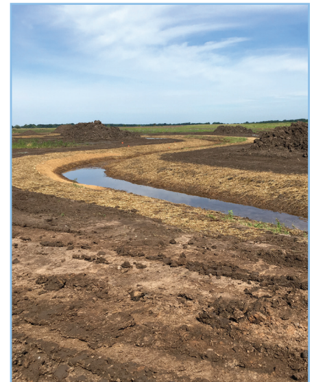
A recreated curve in one local stream. Restoring it to a more natural meandering shape helps improve stream health.
