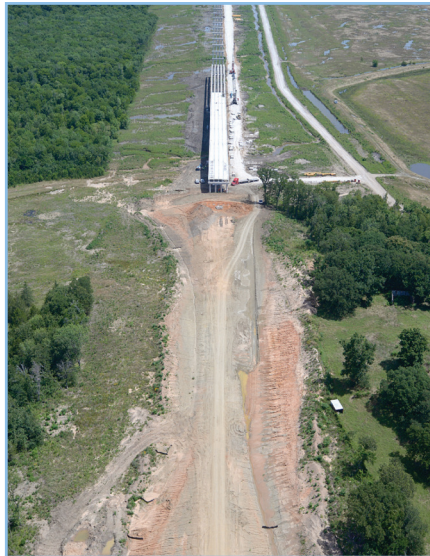
First section of FM 897 taking shape with columns (vertical), caps and beams (horizontal) and deck paneling (one part of driving surface) in place.
