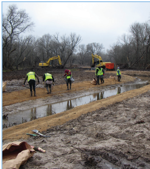
Mitigation workers plant live stakes to restore vegetative support for streambanks.
