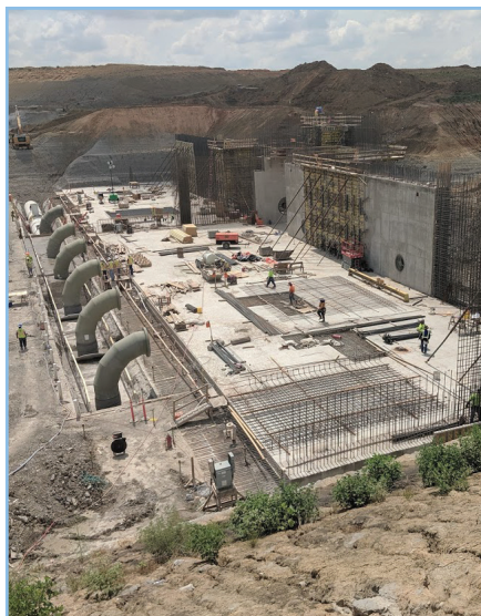
Walls, pipes and pieces taking shape at the lake's raw water pump station.
