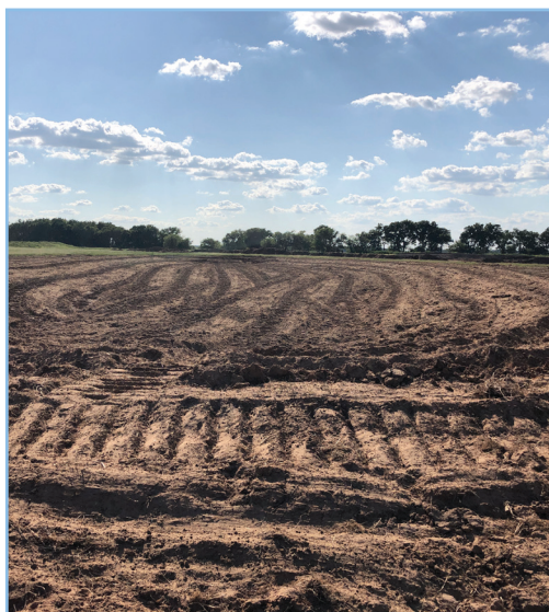
Depressions, berms and ponds constructed for future wetland areas at the mitigation site.
