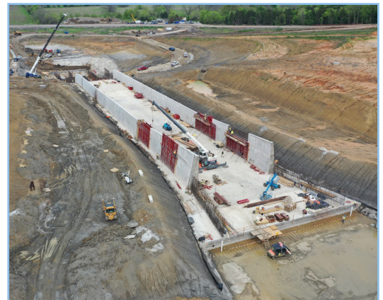
Overhead view of the concrete spillway and walls under construction
