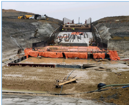
Creating a foundation for the lake spillway
