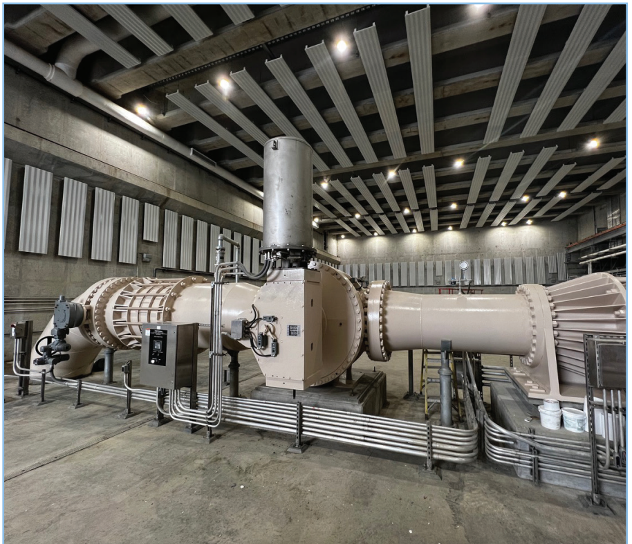
One of the massive pumps in the Raw Water Pump Station, ready to move water out for treatment.
