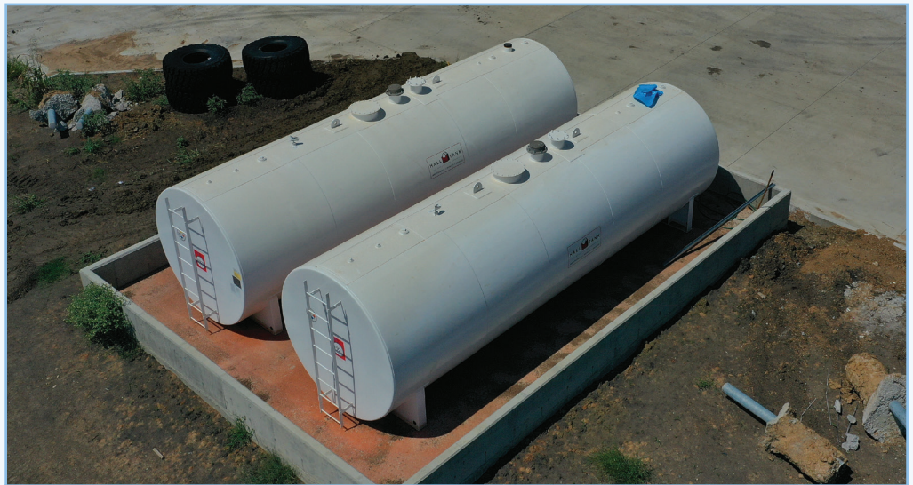
Oxygen is pumped from these tanks and into Bois D'Arc Lake to improve the lake's health.
